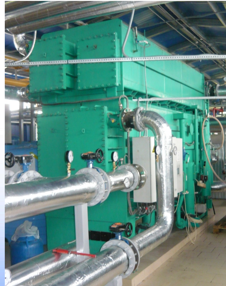
Absorption lithium bromide refrigerating machine (ABHM)
