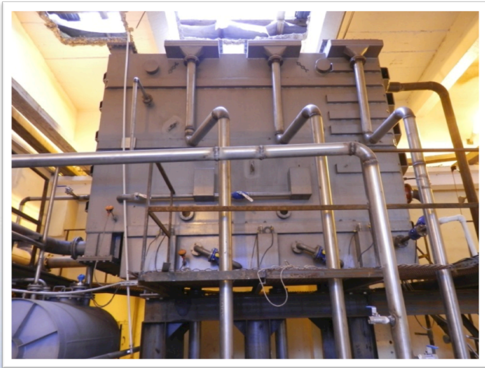
Three-stage plant with a capacity of 7.5 t/h for desalinated water
